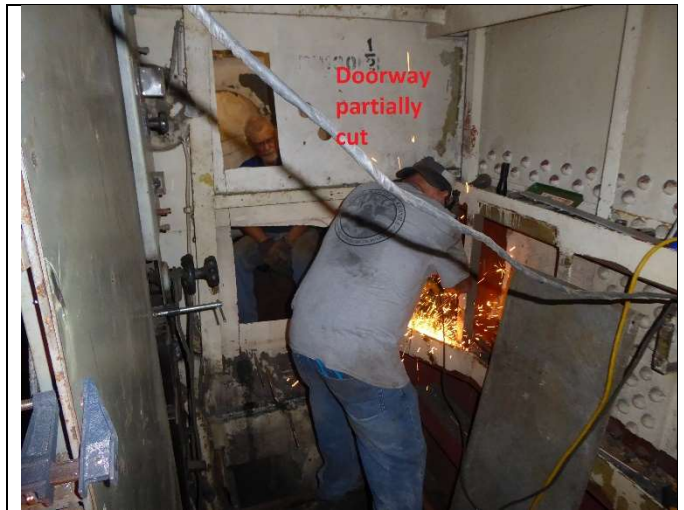
John Hudak watching Ernie Doyle Cut the Doorway
