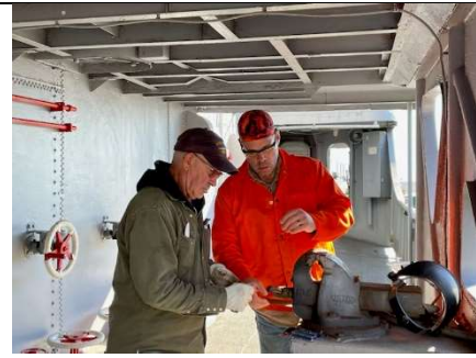
Harry Stoner and Buck Stoner metal fabrication for port side repair.
