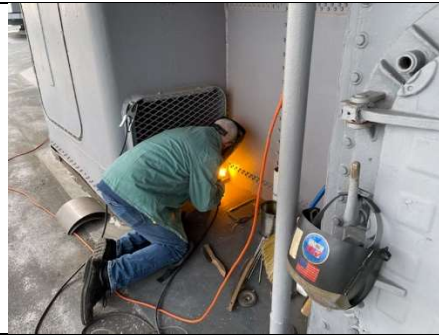
Harry Stoner Welding
