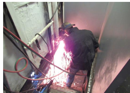
John Hudak cutting access into After Fireroom for visitors soon
