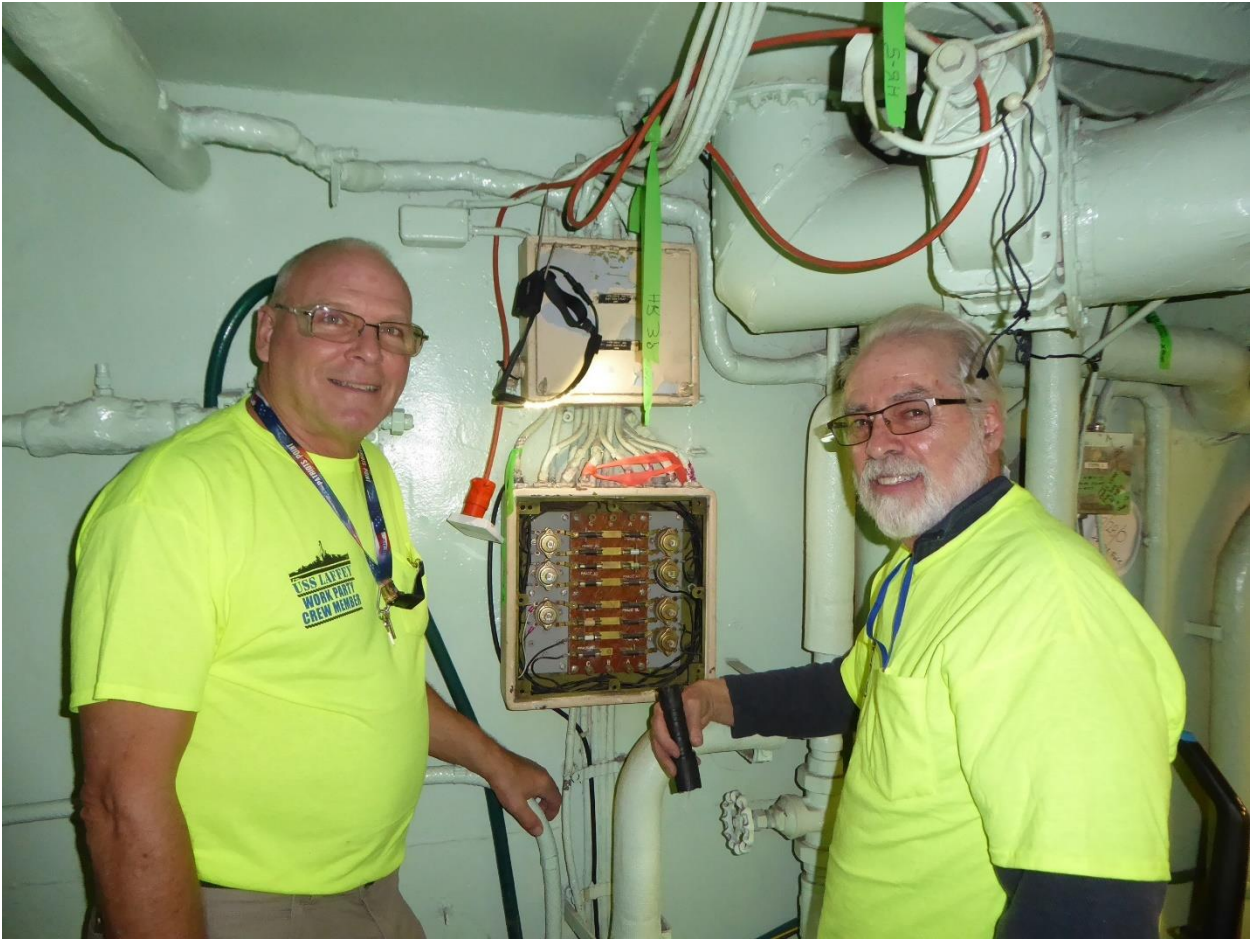
Steve Bade and Marc Jacob repairing Electrical Panel in Chiefs Quarters
