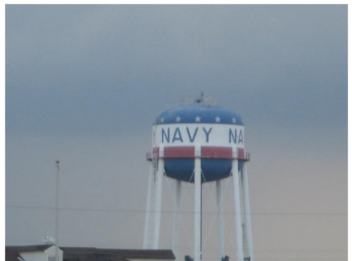
Our very own municipal water tower
