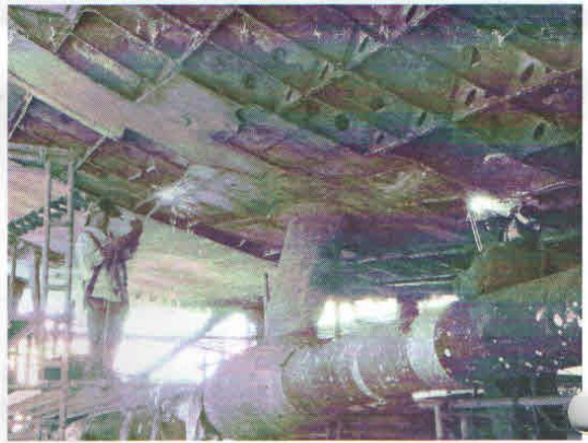
Work being done on the bottom of the Laffey
